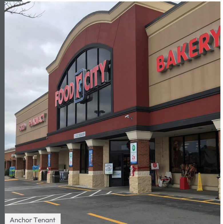
View of storefronts
